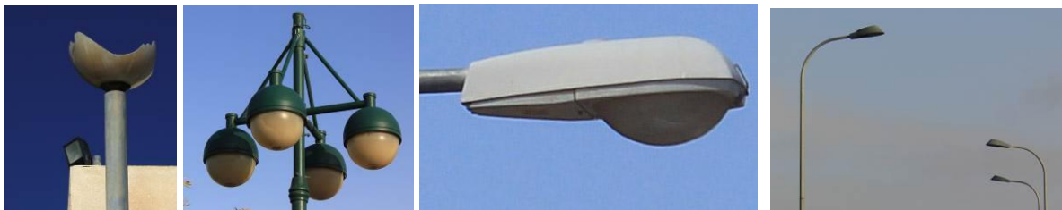
Fig 14: Bad and good (only the right!) oriented luminaires in Mitzpe Ramon
