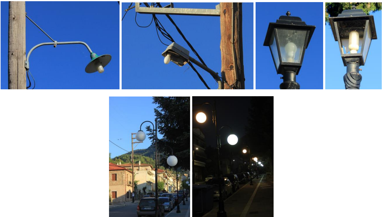
Fig. A6: The luminaires in Kalavrita are very old, inefficient and not very well shielded and waste a lot of light.
